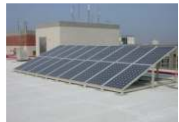
Assembled Solar Panels
